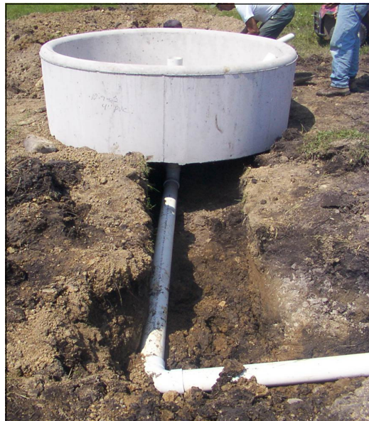
Installation of pipes to a permanent water tank
